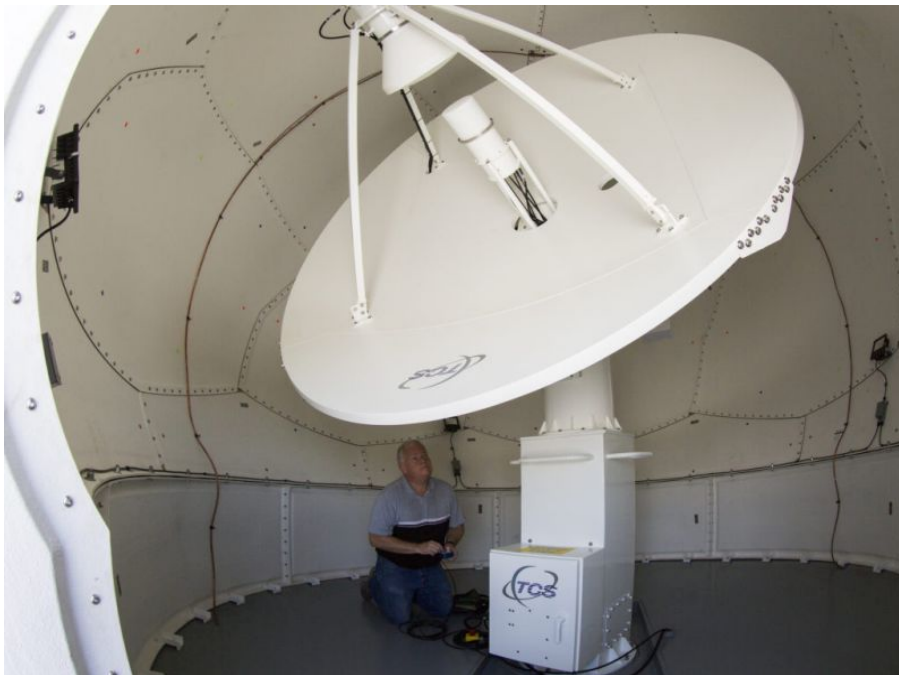
Antenna Inside Radome
